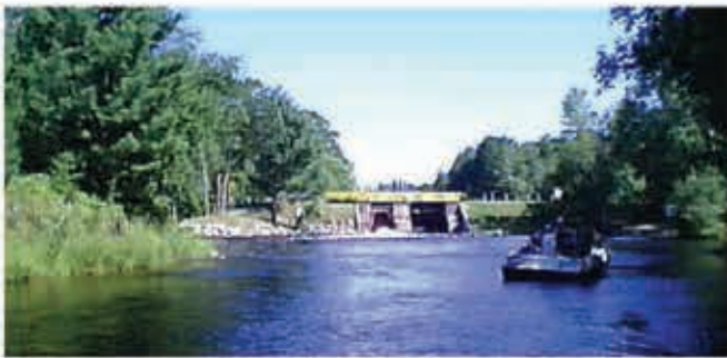
Burnt Rollways Dam viewed from the Eagle River side
